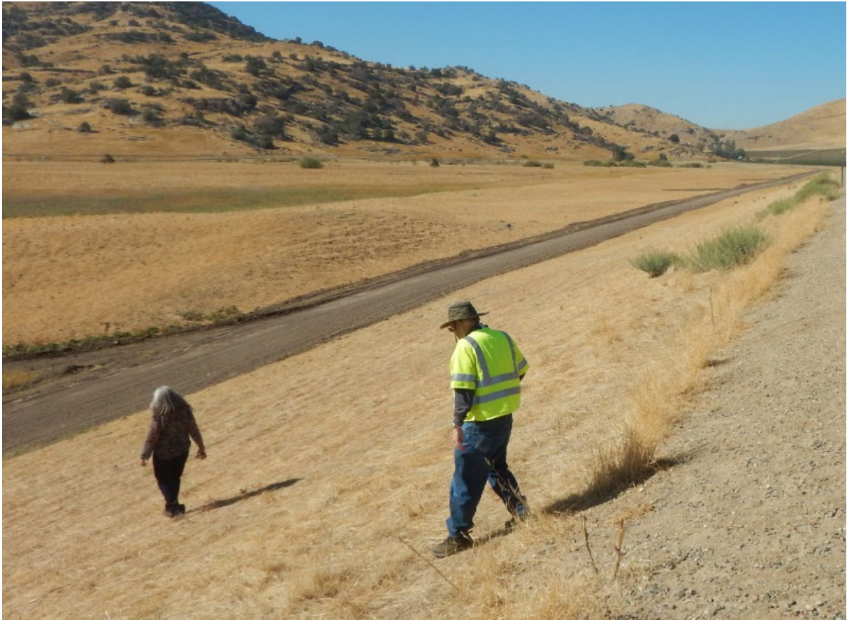
Figure 9. Photo of typical current conditions along Frazier Dike.
